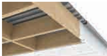
Wooden Structure Underside
